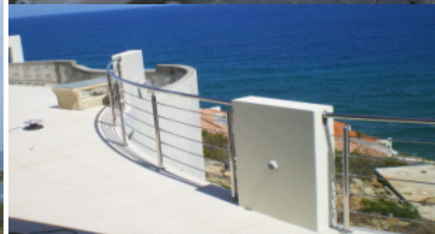
Spiral Staircase and Railing Located: Sant-Matin Island Material: SUS316 and Mirror finish
