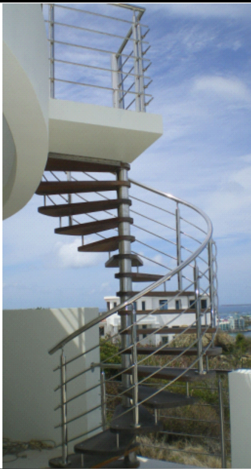
Spiral Staircase and Railing Located: Sant-Matin Island Material: SUS316 and Mirror finish
